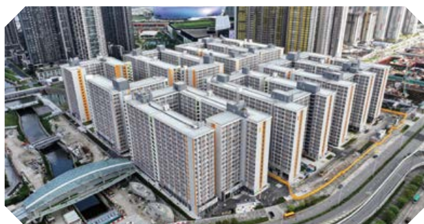
Kai Tak Olympic Avenue Light Public Housing
