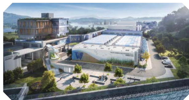
Tseung Kwan O Desalination Plant
